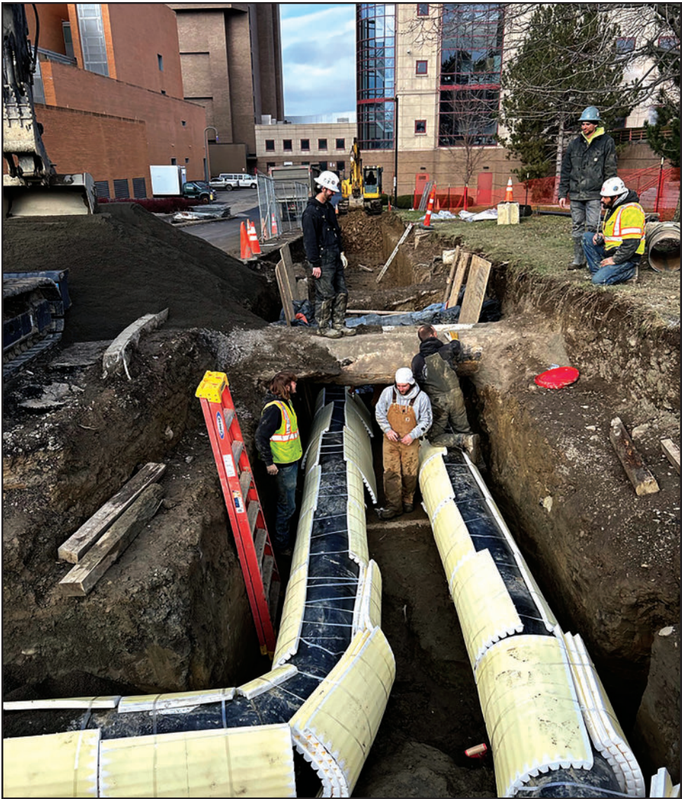
Photo provided New hot water pipes under the sidewalk leading to the Veterinary Medical Center and East Campus Research Facility loading dock area. The new pipes are installed beneath an existing steam line.
